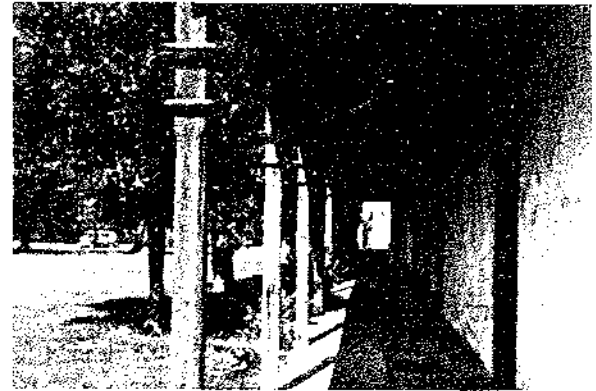
Original posts on porch on front side of the ADOBE.
