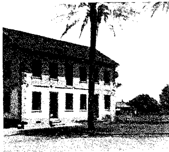
Garnier limestone building -- 1872
